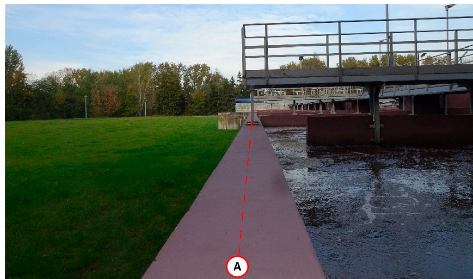
Figure 25. Wall view after repair.
