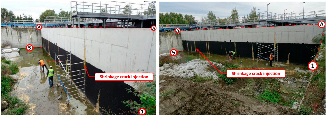
Figure 22. Injection in vertical cracks resulting from concrete shrinkage.
