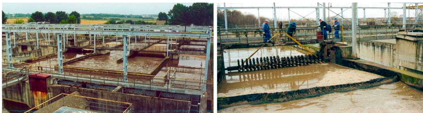
Figure 1. Archival photographs of the biological reactor in the 1990s.
