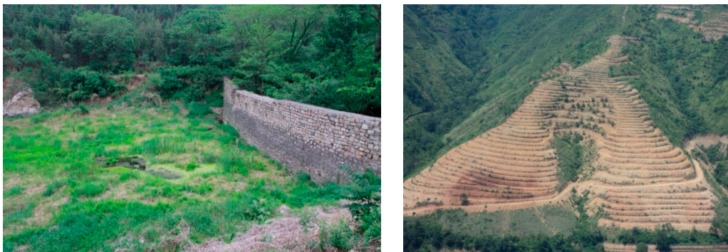
Figure 7. Soil-retaining dam and slopes reshaped into terraces in the Haihe River Basin.
