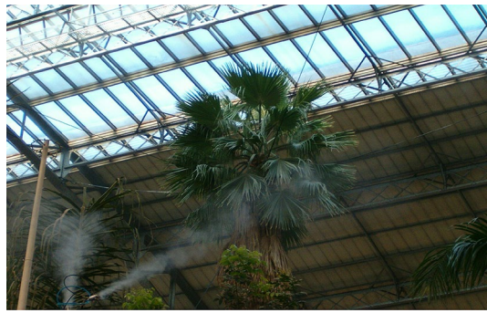
Figure 2. The slender Mexican fan palm anchored to the ceiling of the Atocha train station, Madrid. The cabling configuration was installed to minimise damage in case of post-buckling collapse. The other palms had collapsed before, even though there are no events of wind inside this giant greenhouse.
