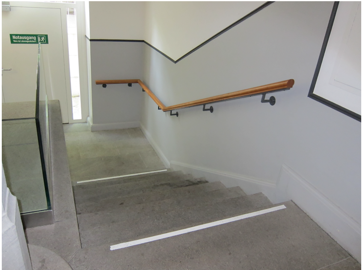
Fig 2. Stairs looking downwards.
