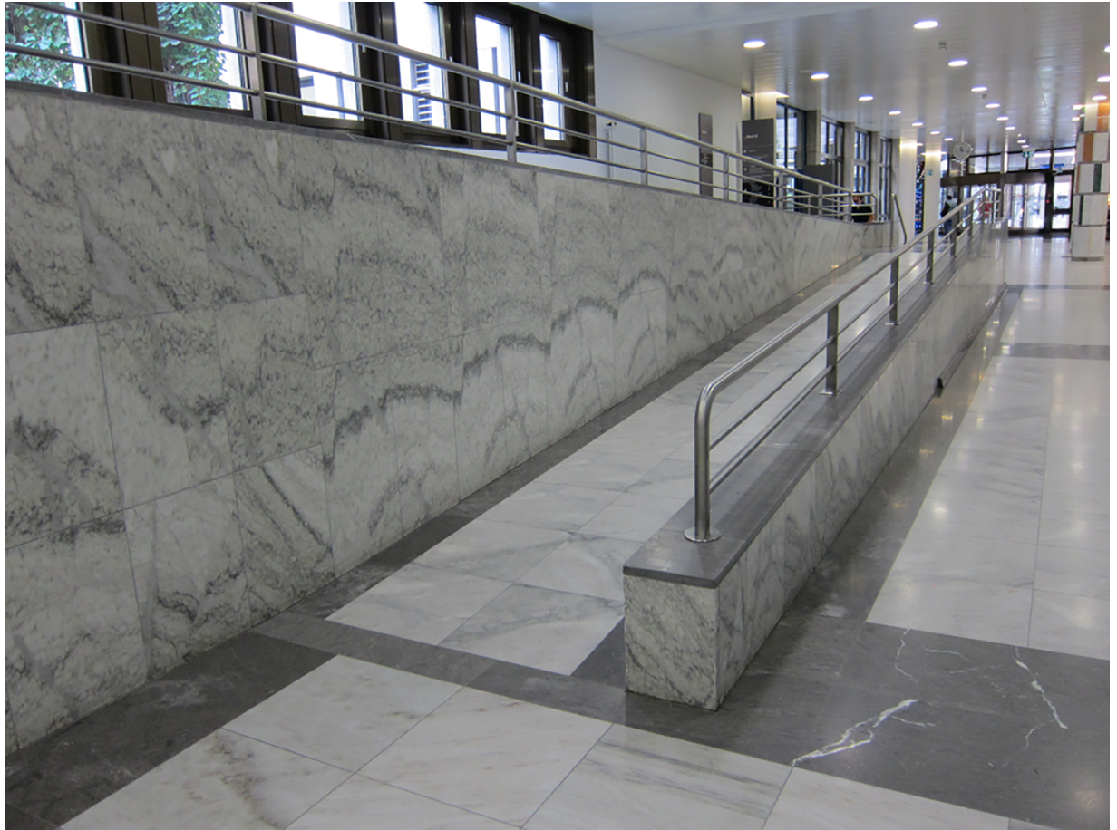
Fig 3. Ramp looking upwards.
