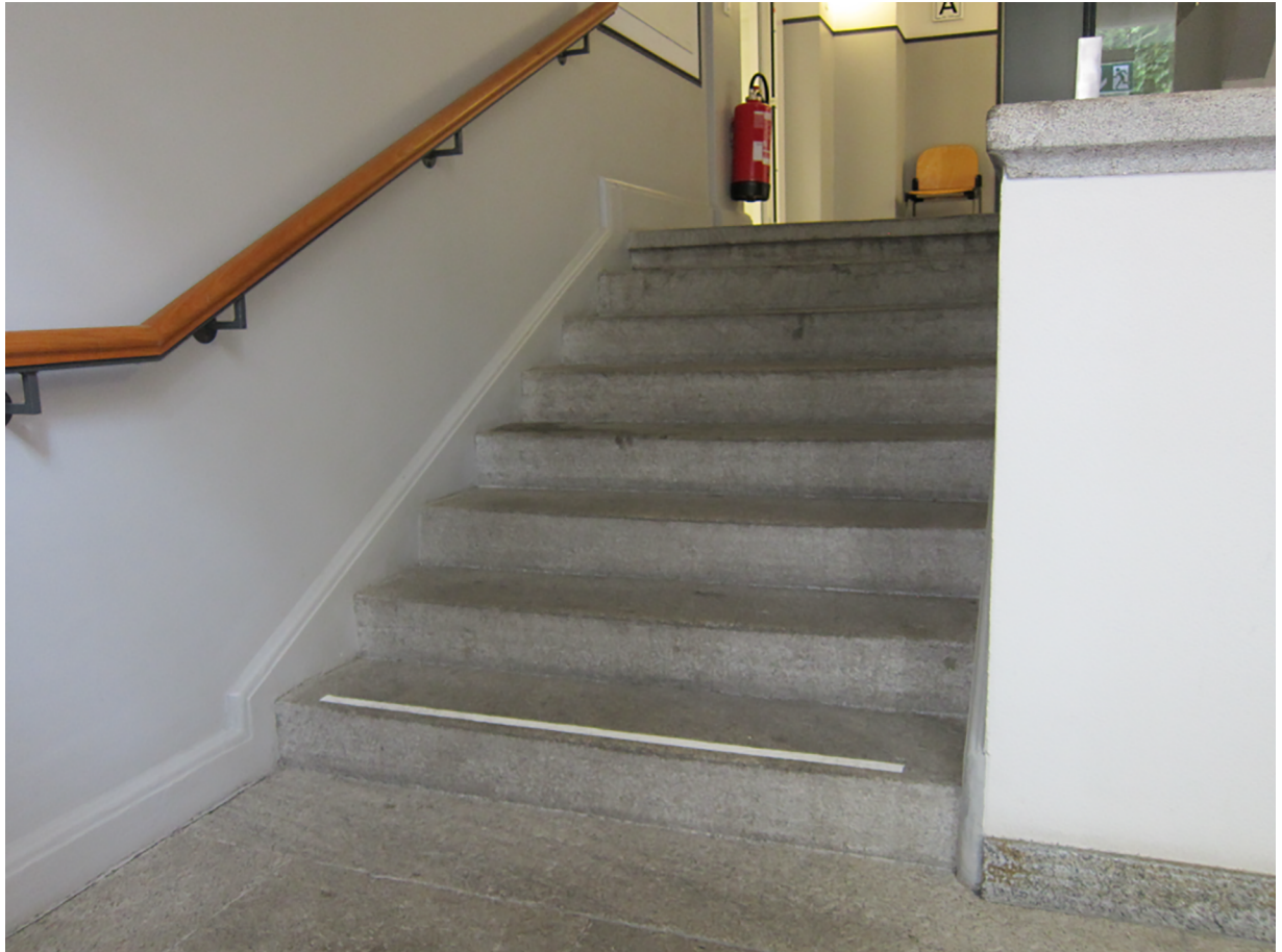
Fig 1. Stairs looking upwards.
