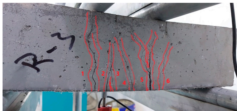
Figure 5. Multi-cracking failure of tested prisms.
