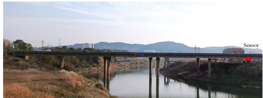
Figure 12. Bridge overview and installation point (red dot) of the inclinometer.
