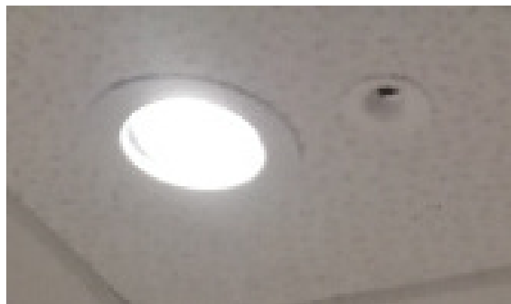
Figure 3. LED lamp and IR sensor mounted on the ceiling.
