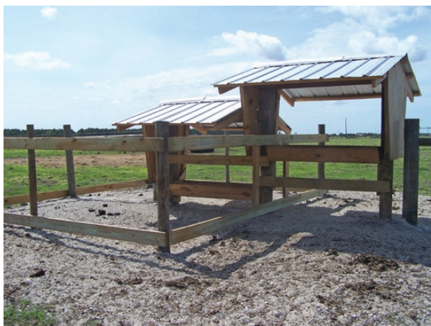
Figure 1. Mineral feeders used in Exp. 1 and 2 were designed to assess mineral intake of cows and calves independent of each other. Calves are excluded by height of the mineral feeder (approximately 100 cm), and cows are excluded by a creep gate restricting entry (approximately 75 cm height). Both feeders are covered by a slanted roof approximately 120 cm above the mineral feeder with the roof edge extending approximately 100 cm from the edge of the mineral feeder.
