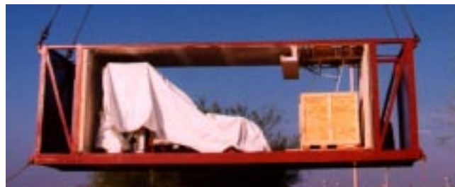
FIG. 3. The central module with the LINAC being lifted into position
