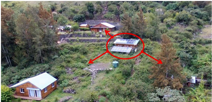
Fig. 3. Aerial view of the microgrid. Battery pack and acquisition devices at the centre, the loads at the three ends.
