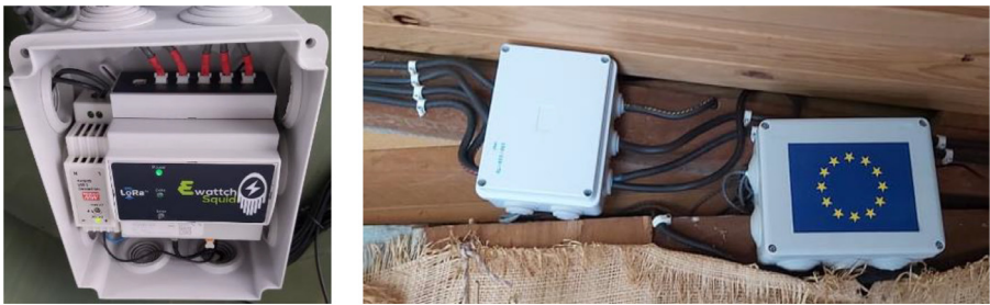
Fig. 6. Consumption recorder: Installation.
