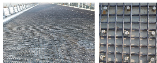
(c) Construction of steel-UHPC composite deck
