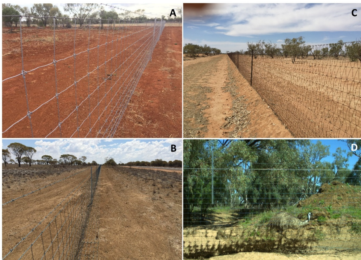
Figure 1. Examples of pest exclusion fence designs on agricultural lands. Examples are of netted cluster fence types in Western Queensland, showing strained aprons with one or two barbed top-wires (A,B) and those without top wires and buried aprons (C). A typical creek crossing is also shown (D), with an excluded emu.
