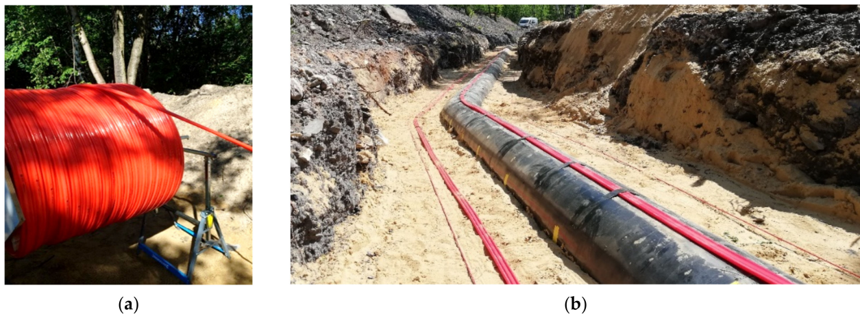
Figure 30. Gas pipeline equipped with 3DSensors: (a) delivery on site in the coil; (b) view of the installed sensors.
