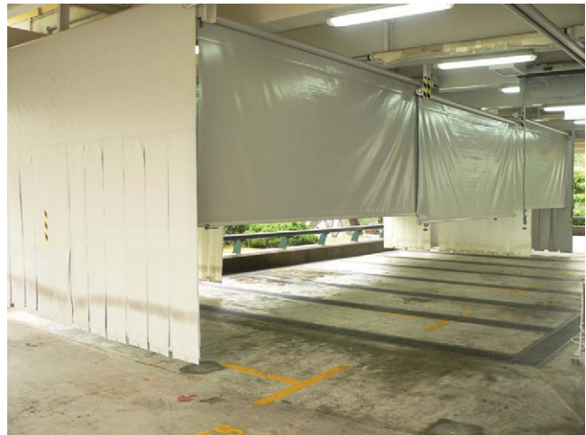
FIGURE 2B-4 A, Fixed immediate deployment decontamination facility at Singapore General Hospital and Drug and Poisons Information Centre. The unit is located in the drive-through ambulance bay in front of the emergency department. This shows the unit in predeployment position. B, Deployment of the unit requires turning on a few switches, which control descent of the shower heads, flexible walls, and temperature control. The unit is ready for operation in approximately 2 minutes. C, Shower heads drop out of the ceiling for self- or assisted irrigation. D, Flexible walls drop from the overhead frame, providing easy ingress, egress, and protection from elements, as well as privacy. E, The unit is ready for use. Floor drains collect the water for appropriate disposal. (Photographs courtesy of Dr. Gaerpo Ponampalam and the Singapore Drug and Poisons Information Centre.)
