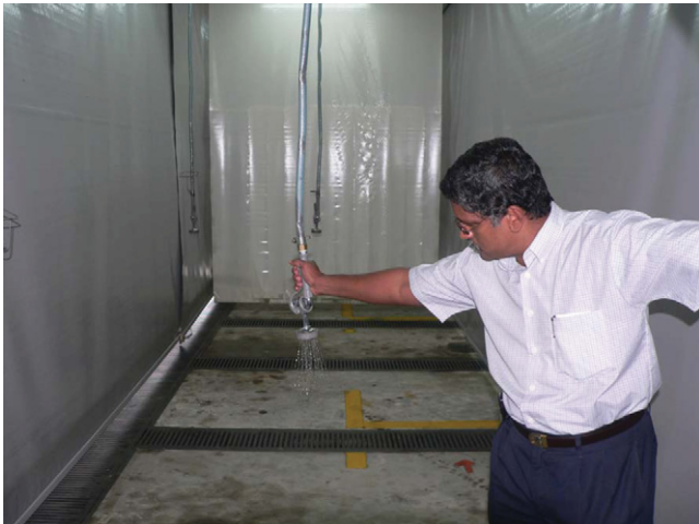
FIGURE 2B-4 A, Fixed immediate deployment decontamination facility at Singapore General Hospital and Drug and Poisons Information Centre. The unit is located in the drive-through ambulance bay in front of the emergency department. This shows the unit in predeployment position. B, Deployment of the unit requires turning on a few switches, which control descent of the shower heads, flexible walls, and temperature control. The unit is ready for operation in approximately 2 minutes. C, Shower heads drop out of the ceiling for self- or assisted irrigation. D, Flexible walls drop from the overhead frame, providing easy ingress, egress, and protection from elements, as well as privacy. E, The unit is ready for use. Floor drains collect the water for appropriate disposal. (Photographs courtesy of Dr. Gaerpo Ponampalam and the Singapore Drug and Poisons Information Centre.)
