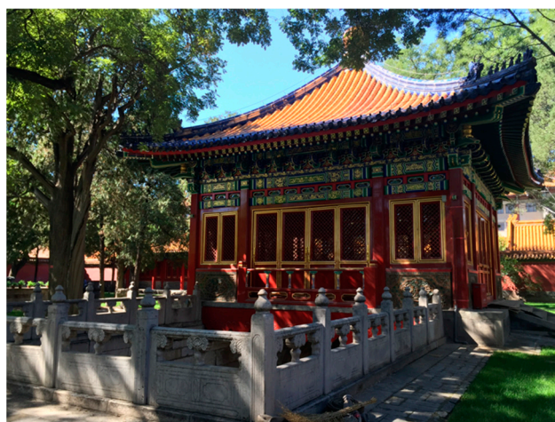
Figure 1. Exterior of Lin'xi Pavilion.
