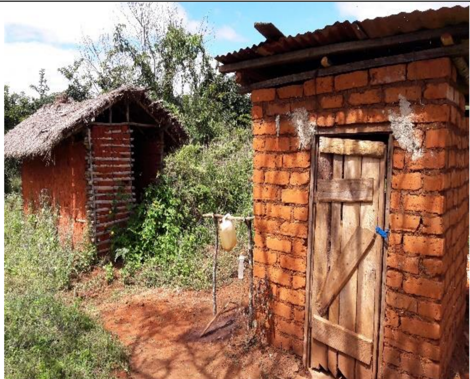
Fig 2. A newly constructed toilet after discarding the old one following the National Sanitation Campaign reported by a household member in Lushoto District, Tanzania.
