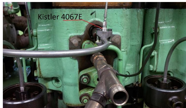
Figure 1. Installation of the Kistler 4067E injection pressure sensor (in the background, the electric cable of the Kistler 6353A24 combustion pressure sensor protruding from the indicator cock).
