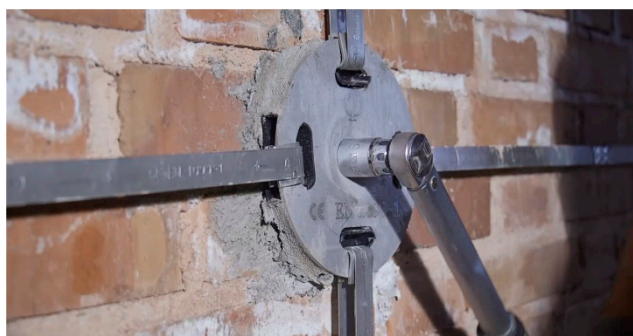
Figure 14. Tightening of a threaded bar [54].
