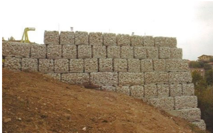
Figure 22. Metallic gabions for retaining walls and slope stabilization.
