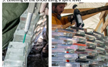
7. Dispensing of 3M DP610 (left) and of the Fast-curing experimental Dowsil Adhesive (right).
