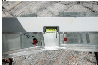
5. Levelling of the bricks using a spirit level
