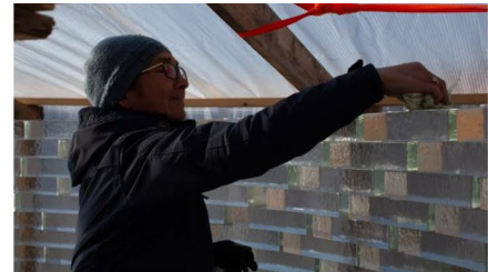
2. Bricks of the bottom layer are cleaned
