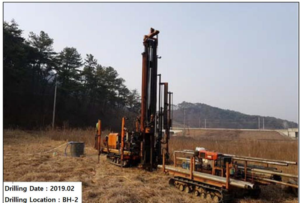
Figure 15. Rotary drilling rig using the NX-size core barrel ( $\phi 76$  mm).
