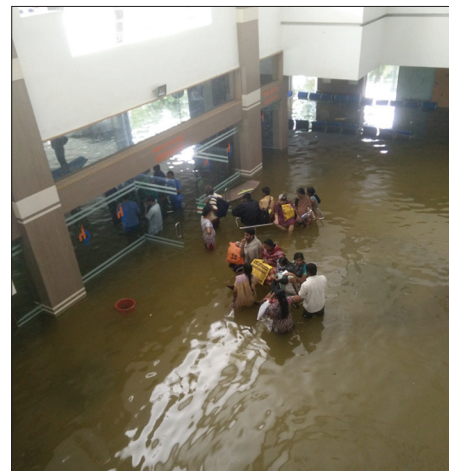
Figure 4: Picture taken inside the main hospital building at the time of evacuation
