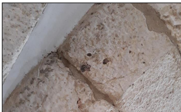
Figure 12. Silica (dark spots) found in an ashlar of the Tower of Belém.
