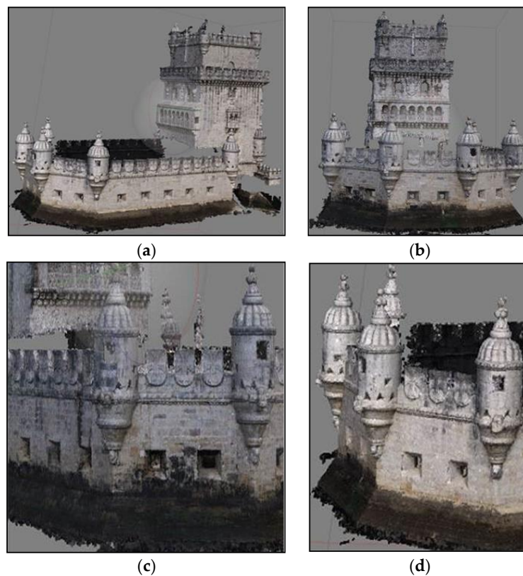
Figure 5. Photogrammetric 3D point cloud: (a) East wall; (b) South wall; (c) and (d) Details of the South wall.
