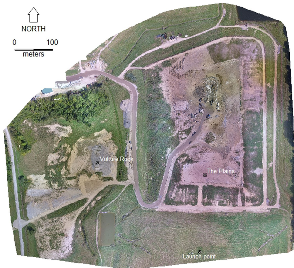
Figure 1. Study locations at the Erie County Landfill, Milan, Ohio. Base map was created using geo-referenced images from the DJI Inspire and Drone2Map (version 1.3.2.232, ESRI, Redlands, California, USA). Map was created by M.B.P.
