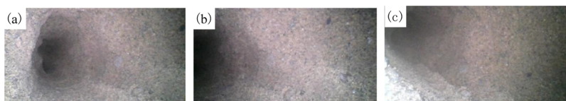
Figure 13. No. 2 borehole peeper. (a) Surrounding rock in the upper region, (b) surrounding rock in the middle region, and (c) surrounding rock in the lower region.
