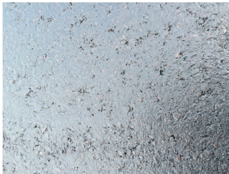
Figure 6. Effect of paving using the high-modulus asphalt mixture.
