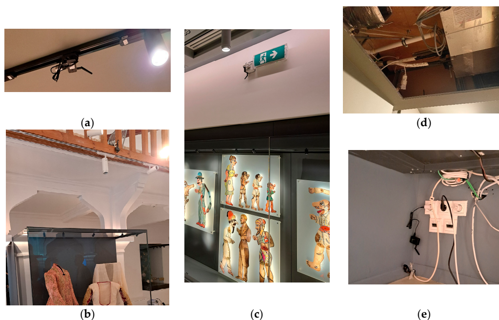
Figure 4. BLE gateway installation types in the MNEP: (a) ceiling lightning bars (ERCO), (b) mounted on wooden bars, (c) wall-mounted on emergency light, (d) within false ceiling, and (e) under the showcase.
