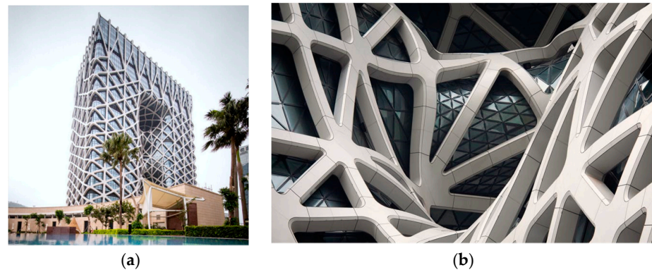
Figure 1. The Morpheus Hotel in Macau: (a) overall shape of building, (b) various joint configurations.
