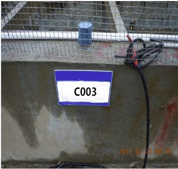
Fig. 11. Diaphragm wall horizontal displacement monitoring point C003.
