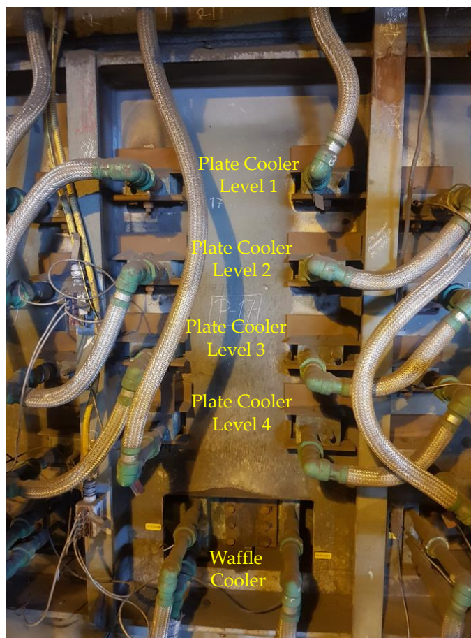
Figure 6. External view of panel #17 of the 72 panels wallside that radially compose the furnace.
