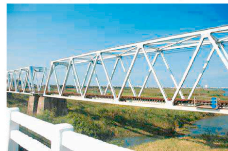
h) Simply support steel truss
