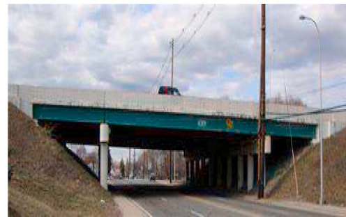
f) Simply support steel plate girder
