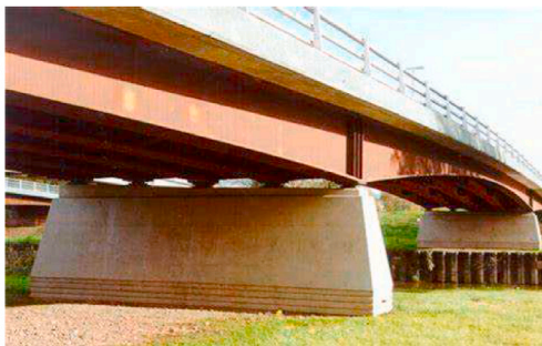
e) Continuous steel plate girder
