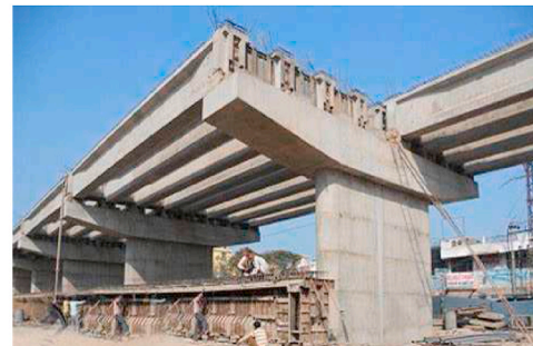
b) Pre-cast PT beams
