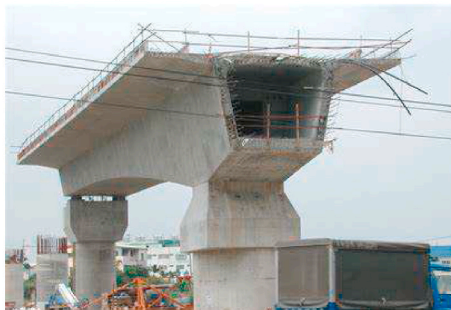
c) Cast in situ RC box section
