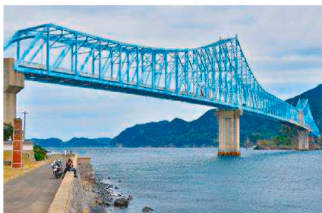
g) Continuous steel truss
