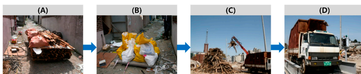
Figure 1. The data collection methods for WGR calculation: (A) Generated CW; (B) CW Type Classification; (C) Loading Dump Truck; (D) Weight Measurement.
