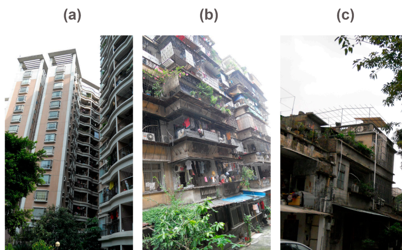
Figure 2. Types of residential buildings in the 2014 Guangzhou outbreak (from left to right: (a) high-rise modern apartment; (b) old flat; (c) shed).
