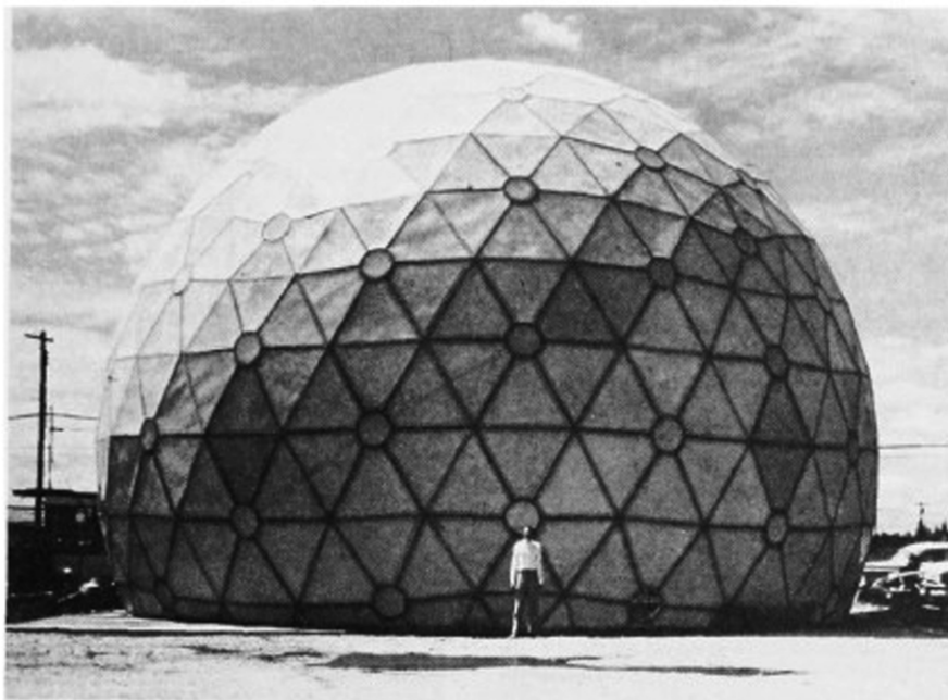
FIGURE 5. A Fuller geodesic dome (Radome designed by Geometrics, Inc., Cambridge, Mass.). Note that the surface is made up of quasi-equivalent triangles and that these are grouped in hexamers and pentamers about the small rings of the dome. (Photograph supplied by W. H. Wainwright).
