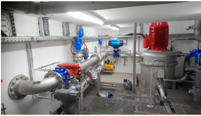
Figure 7. Counterpressure Pelton turbine, photo courtesy of Hirschi Lukas (Haeny company).
