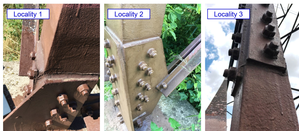
Figure 18. Functional crevice protection with sealant (selected examples).
