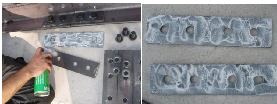
Figure 9. Application of Teflon Vaseline to the splices.
