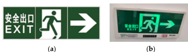
Figure 1. The current color combination of safety sign in China. (a) “Green and white”, from Chinese GB 13495.1-2015 ( Fire Safety Signs-Part 1: Signs ), and Chinese GB/T 23809-2009 ( Safety Way Guidance Systems-Setting Principles and Requirements ), etc.; (b) “Green and black”, the real visual effect after charging in Zhengzhou Zijing Mountain subway station and the other subway stations in China.
