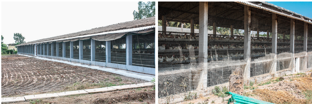
Figure 1 Layer parent farm (a) and commercial layer farm (b) in India. Both are multiage farms with natural ventilation and curtains. Note the clean environment and cement borders around the building in (a) in contrast with the commercial farm with plants growing up to the building and junk lying around in (b).
