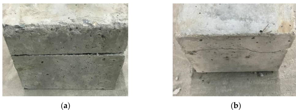
Figure 4. Shear failure mode of the recycled aggregate concrete for: (a) surface of the concrete specimen along the vertical shear direction; and (b) surface of the concrete specimen along the horizontal shear direction.
