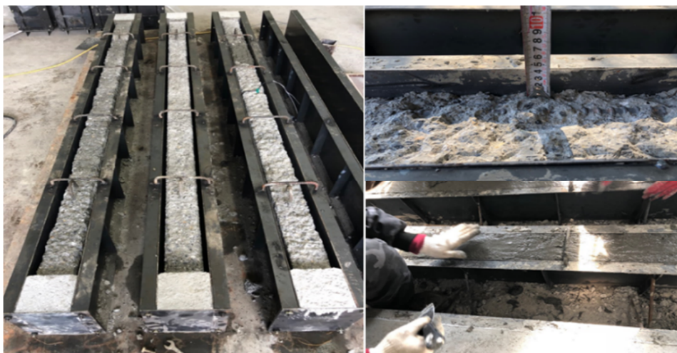
Figure 3. Strengthening process using chiseling and NSHSDC cast in situ strengthening technique.
