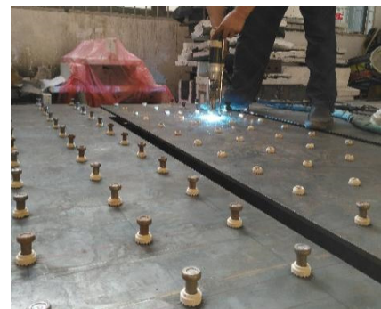
(b) Welding studs
