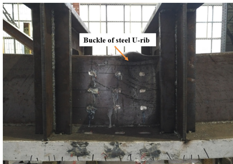
(a) Crack distribution in the lateral direction
