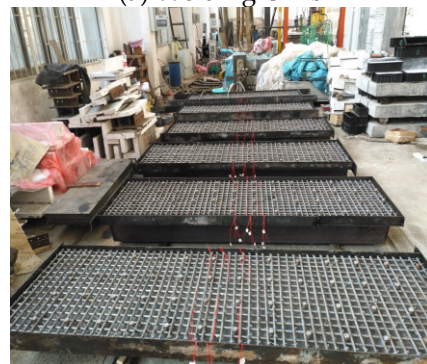
(c) Binding reinforcement
