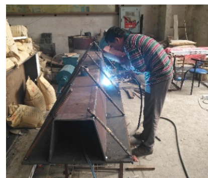
(a) Welding U-rib
