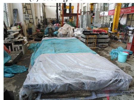
(f) Steam curing of UHPFRC
