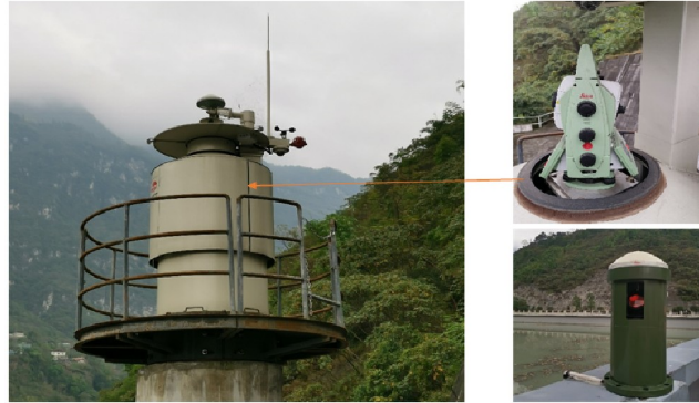
Fig 1. Dam deformation monitoring system based on robotic total stations.
