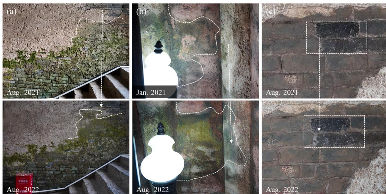
**Fig. 10.** Microbial growth in two tombs from 2021 to 2022: (a) the west wall in the entrance chamber of the Shunling Tomb; (b) the east wall in the middle chamber of the Qinling Tomb; (c) the west wall in the middle chamber of the Shunling Tomb.
