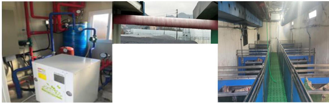
Figure 2. Schematic diagram of the geothermal heat pump (GHP) system for the pig house.
