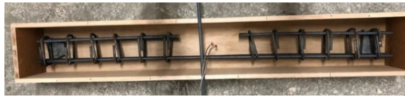
Figure 3. The configuration of the steel rebar and thermocouple.
