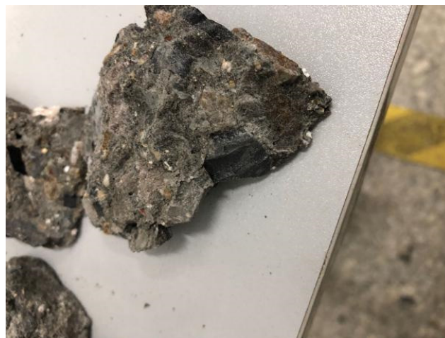
Figure 5. Damaged concrete fragments.
