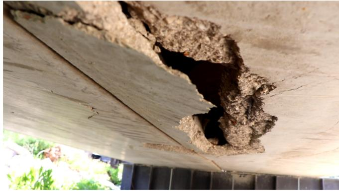
Figure 8. Closed view for the structural damage in hollow core slab from the first impact.
