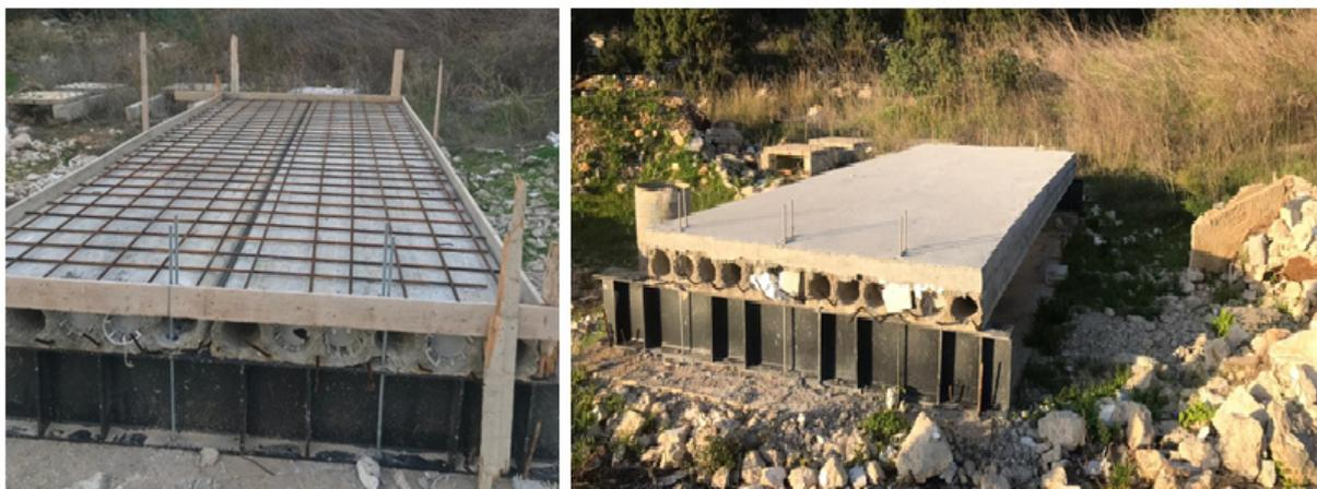
**Figure 2.** Single span hollow core slab with concrete topping site execution.
