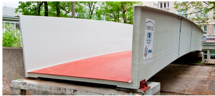
Figure 1. Composite footbridge designed within the FOBRIDGE project.
