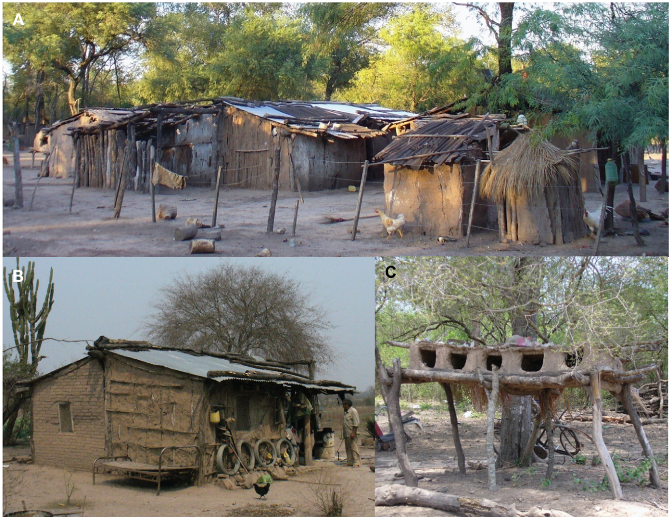
Figure 2. Typical structures of rural Pampa del Indio. A: Domicile and part of peridomicile exhibiting a variety of roof materials (corrugated metal and tarred-cardboard sheets, and thatch). B: A domicile, partly with mud-stick walls, partly with walls made of brick laid on mud, and a corrugated metal roof. C: A mud 'nidero' where chickens and other poultry nest. doi:10.1371/journal.pntd.0001349.g002
