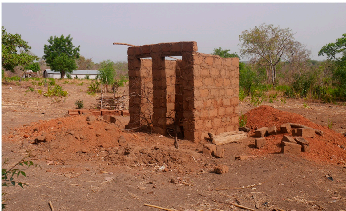
Figure 2. Pit is dug and superstructure constructed.
