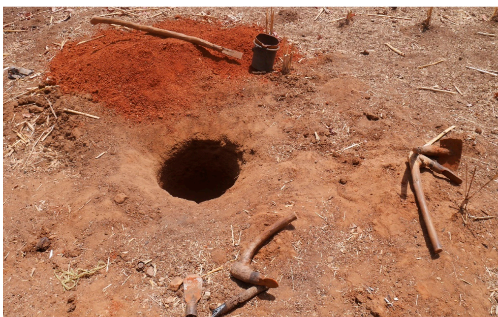
Figure 1. Only pit is dug.
