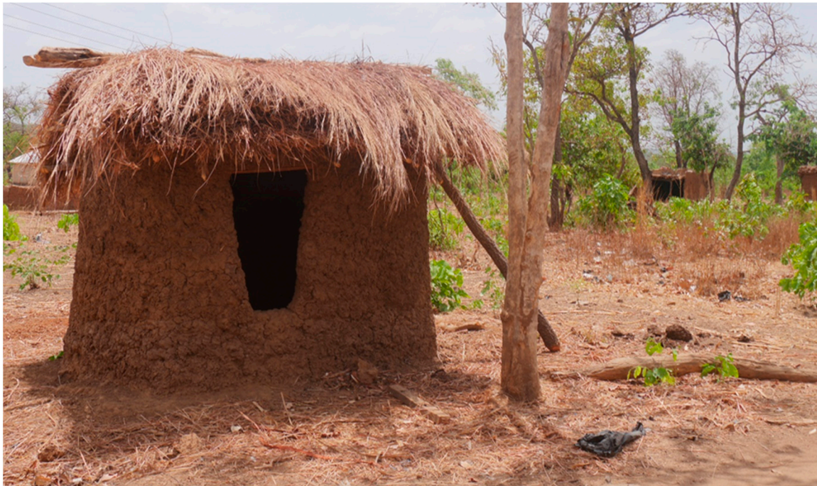
Figure 3. Pit is dug, superstructure constructed and latrine is roofed.
