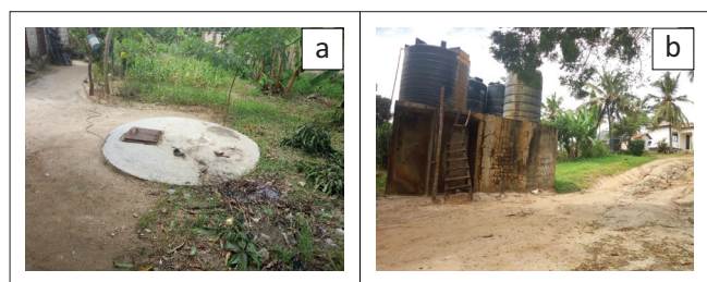
FIGURE 3: (a) Storage tank on the ground surface, (b) Overhead storage tank much safer than ground storage tanks which are risky.
